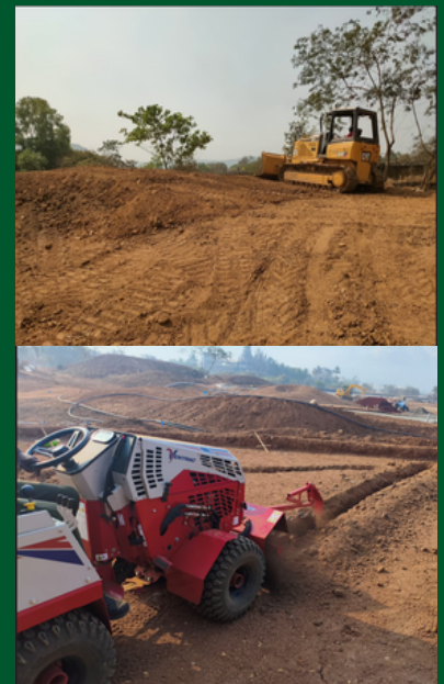
Equipments used for constructio activities
